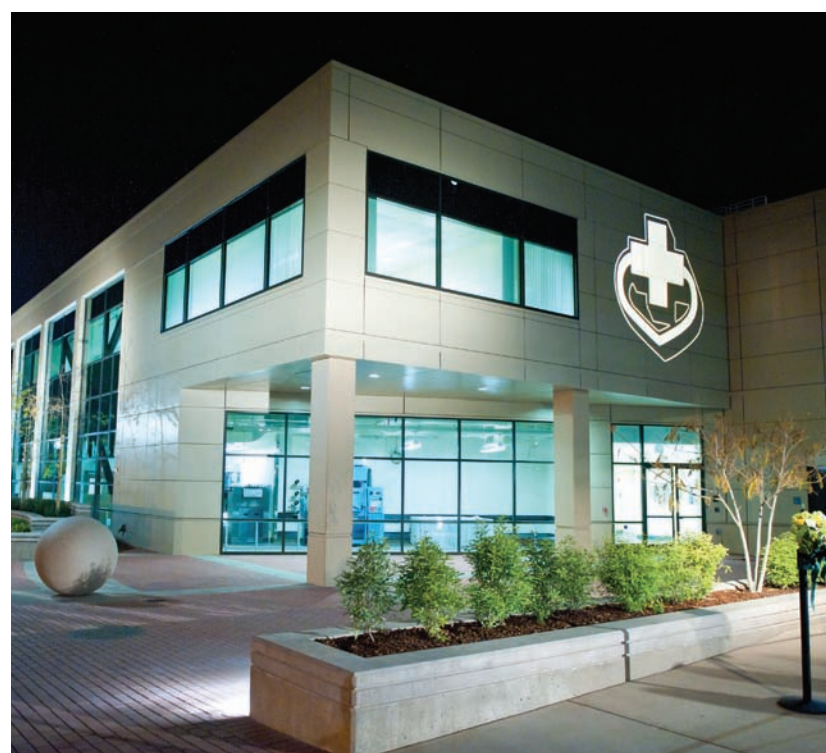
The new Central Utility Plant, completed in December 2011, provides energy- and cost-efficient systems for operating the hospital.
