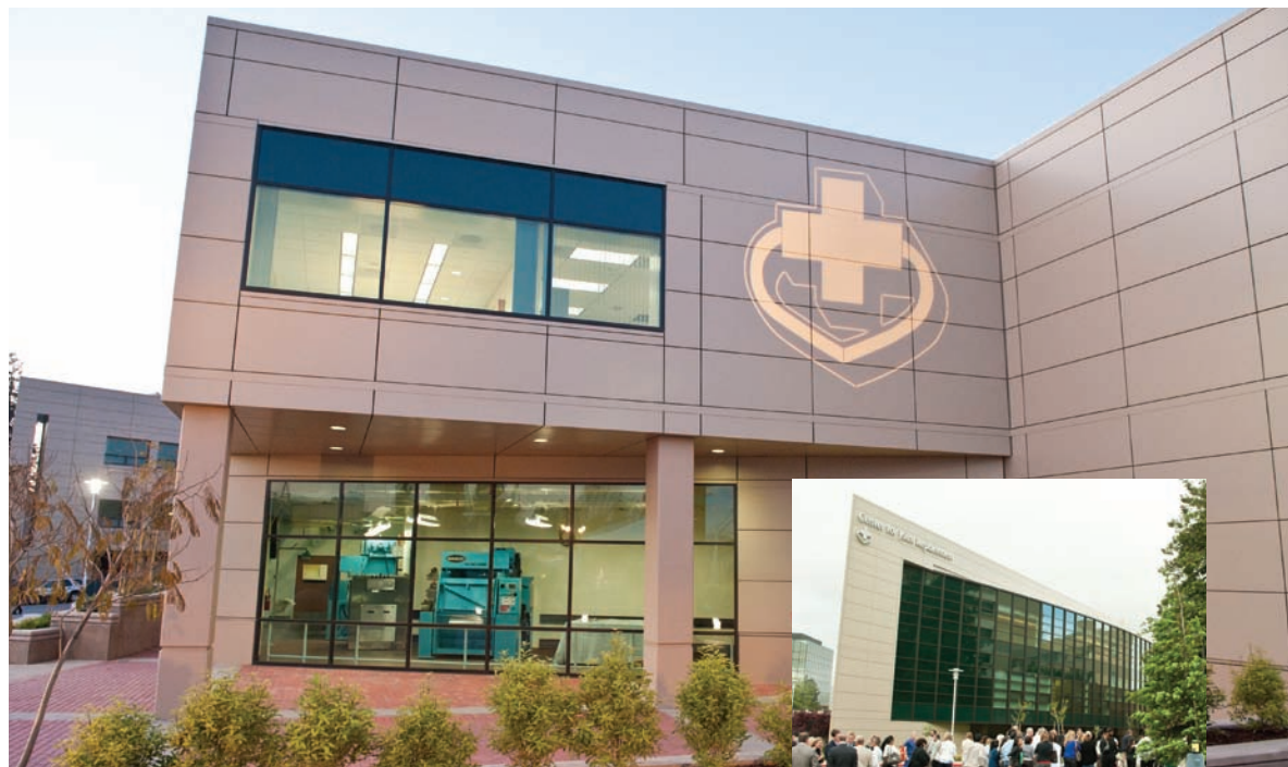
The 37,000-square-foot Central Utility Plant now supplies all the necessary utilities to existing facilities and will support all functions of Washington Hospital's campus of the future.
